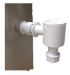
Fig. 1.3a, Showing mains water connection showing combined isolating valve and flow limiter installed & b, Quick release filter attached to overflow warning pipe (supplied loose).
