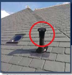
Poly-Air installed on a roof ventilation pipe.
