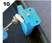
Place the ballcock support over the location post and bracket section over the side wall of the trough.
