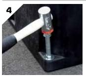
The anchors should be a tight fit and will need to be driven home with a mallet.
