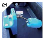
Once tightened bring the float valve back to its vertical alignment position and secure the ballcock cover again.
