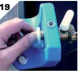
Remove the ballcock cover to gain access to the float valve. Loosen the nut so that it is 3-5mm from the support wall.
