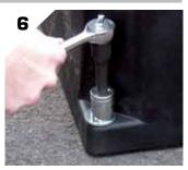
Tighten the anchors to 22.0Nm torque for concrete. Tightening will fan out the bolt sheath in the hole holding it secure.
