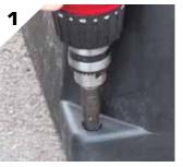
Locate the 4 ground fixing holes at the 4 corners of the trough. Place the drill through the holes and spot drill the locations.
