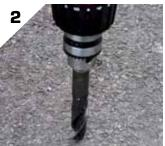
Using a 16mm diameter masonry drill bit, drill 4 holes to a depth of 110mm and remove debris from holes.
