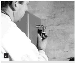
Connect overflow to compression warning pipe assembly ensuring warning pipe accommodates incoming supply.
