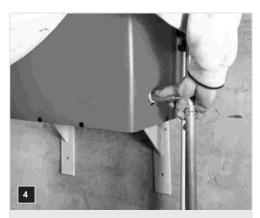
Connect outlet into 22mm push fit tank connector. This push fit tank connector accomodates both 22mm copper and 22mm plastic pipe.
