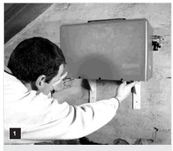
Remove tank from box and put onto a pair of heavy-duty brackets or across ceiling joists.
