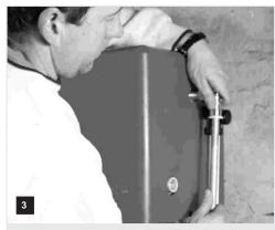
Connect incoming cold feed into the push fit service valve. This push fit service valve accommodates both 15mm copper or 15mm plastic pipe.
