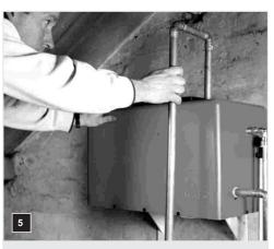
Remove expansion pipe cap and fit 22mm expansion pipe through rubber grommet.
