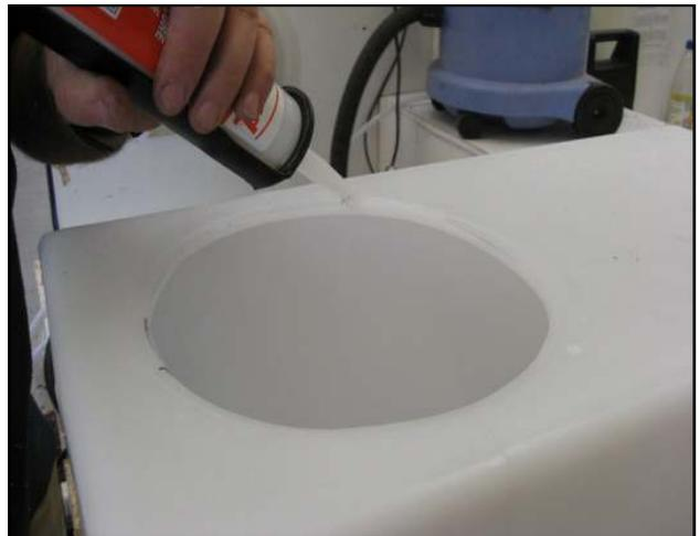
Remove the neck ring, run a bead of silicone around hole on tank.
