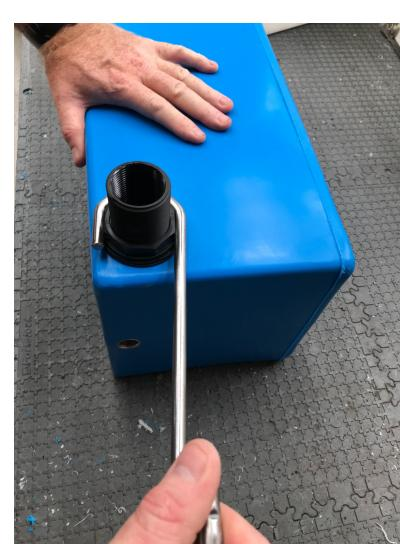
Tighten the back nut using a suitable tool, be careful not to damage the thread.
