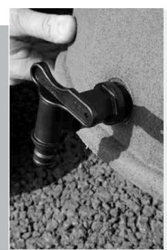
4 Screw the Polybutt tap, clockwise, into the outlet hole. When the tap is fully secured the 'off' valve should be positioned at the top with the outlet of the tap pointing downwards.
